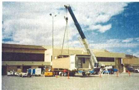
**Ticket Counters Moved**—We moved the ticket counters 8' into the lobby to relocate the TSA checked baggage inspection behind the check-in process. This greatly improved customer service and allows for continued proliferation of self service check-in devices.
